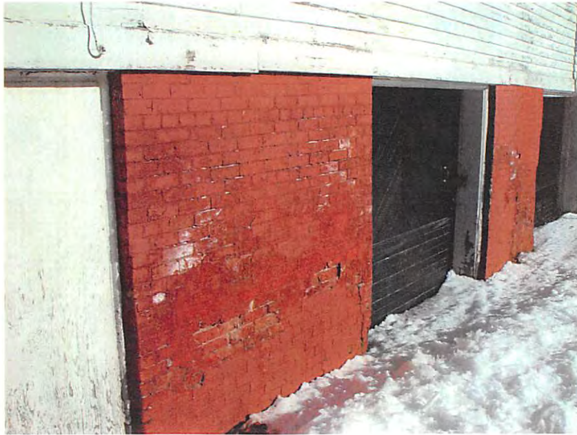
Right Side Brick Foundation
