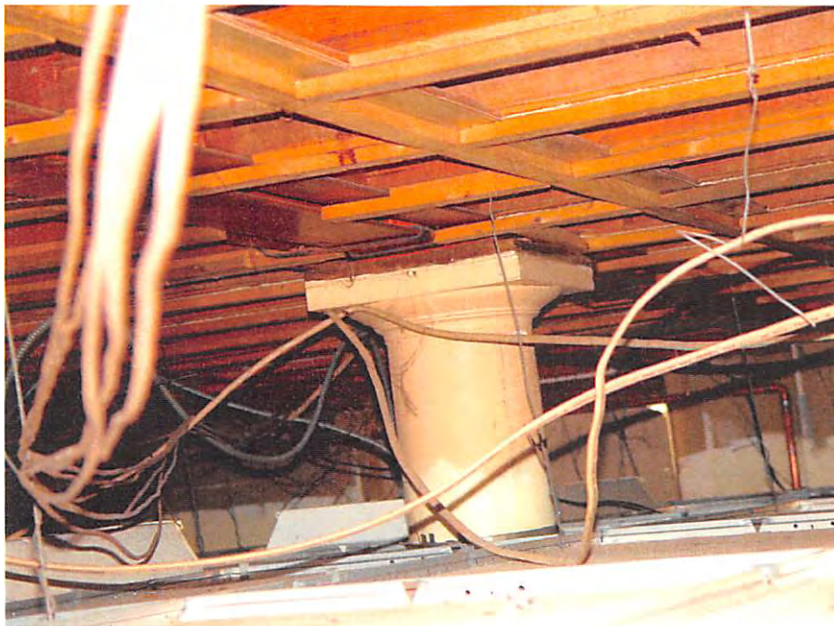
Second Floor Framing
