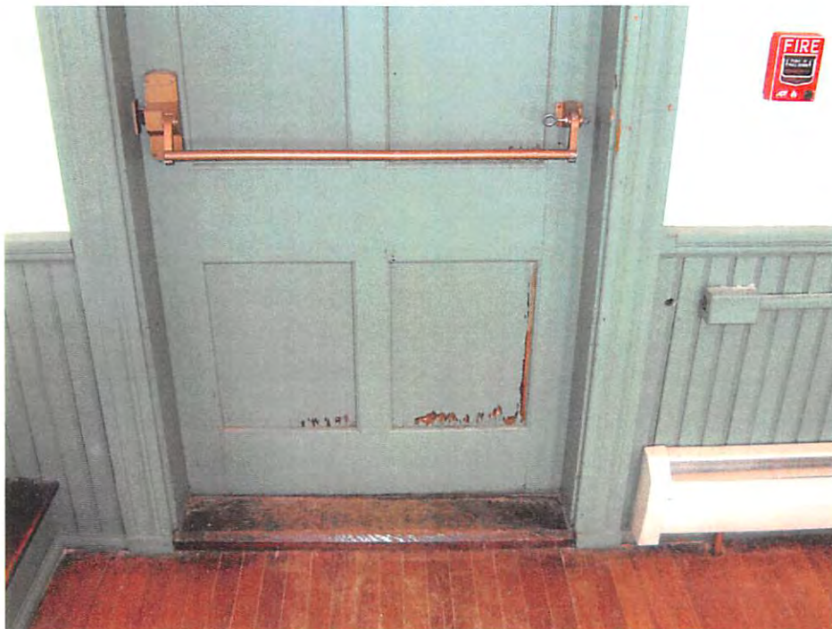
SECOND FLOOR FIRE ESCAPE EXIT DOOR
