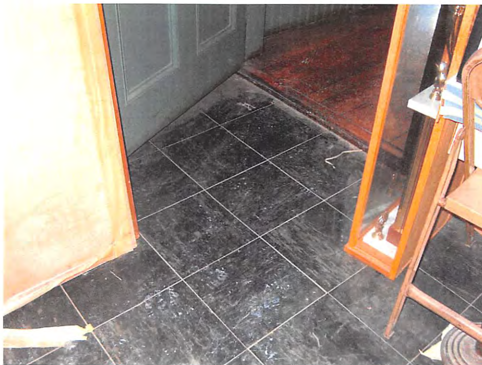
SECOND FLOOR OFFICE
