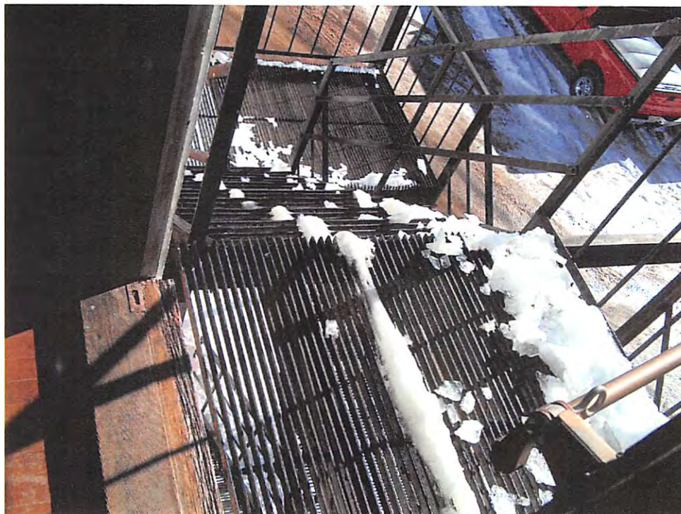
SECOND FLOOR FIRE ESCAPE
