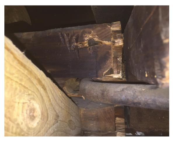
The engineer, Peter Reynolds, reviewing the damaged area has suggested back to back steel channels surrounding and supporting the existing rafter with welded plates for existing tie rod. This is similar to the 2012 study which called for steel I-beams supporting all existing rafters with steel collar ties. The Committee agrees conceptually with the method of reinforcement but believes that a better alternative to steel reinforcement would be laminated veneer lumber (LVL¹).
