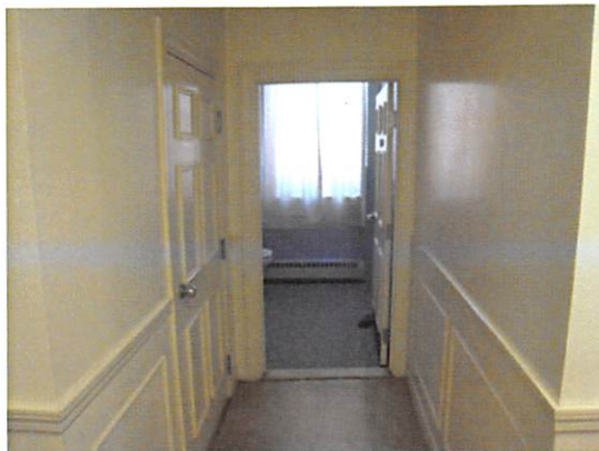
Left: Paneled wainscot and doors. Right: Greek Revival door casing characterized by channels and round corner medallion.
