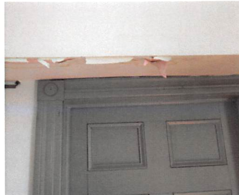
Left: Paneled wainscot and doors. Right: Greek Revival door casing characterized by channels and round corner medallion.
