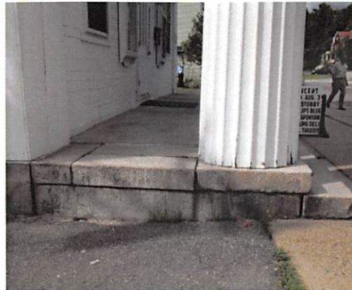
Left: Fluted wood column resting on granite porch at portico. Right: 12 over 12 sash configuration.
