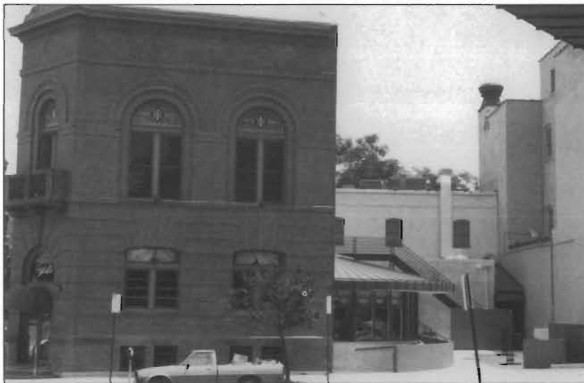
The historic residence is on the right. By copying the decorative gable and three-part window in the new addition, the old and new portions are virtually indistinguishable. This approach violates the Standards for Rehabilitation.
