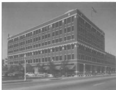
When the six-over-six windows were replaced with inappropriate single sheets of tinted glass, the historic industrial character of this building was lost.
