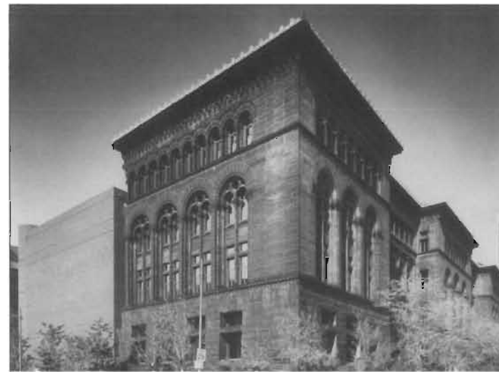
A new 10-story wing added to the back of a historic library constitutes major expansion, yet is compatible because it reads as a subsidiary unit to the much larger historic building.
