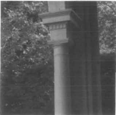
To replace deteriorated portions of the column, strips of new wood were milled to conform to the shape and appearance of the old column framework, glued in place, then back-primed and painted.
