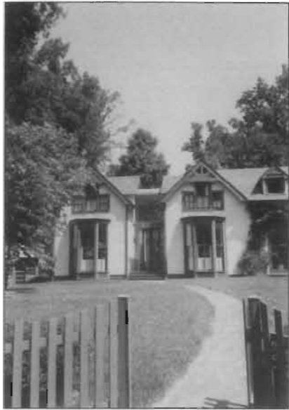
The historic residence is on the right. By copying the decorative gable and three-part window in the new addition, the old and new portions are virtually indistinguishable. This approach violates the Standards for Rehabilitation.
