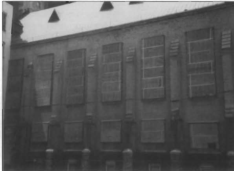
▲► The roof and stained glass windows of this historic church have been appropriately covered with plywood as a protective measure during construction of a new building on an adjacent lot.
