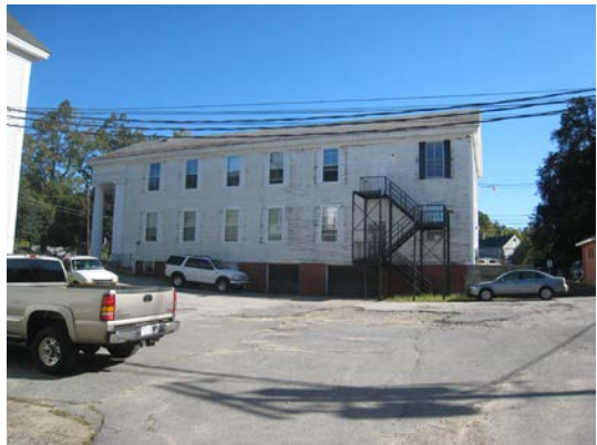
Parking lot on west side.
