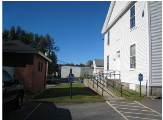
Brick fire proof storage building and concrete ramp at south side of building.
