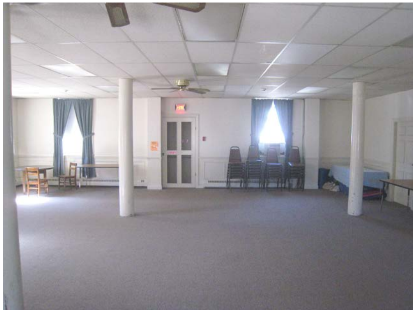
First floor: View south toward exit door in Recreation Room. Note wood columns from the 1893 addition which help support the large Assembly Room, carpeting and dropped ceiling.
