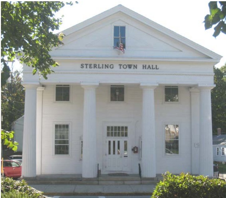
Facade (north elevation).
