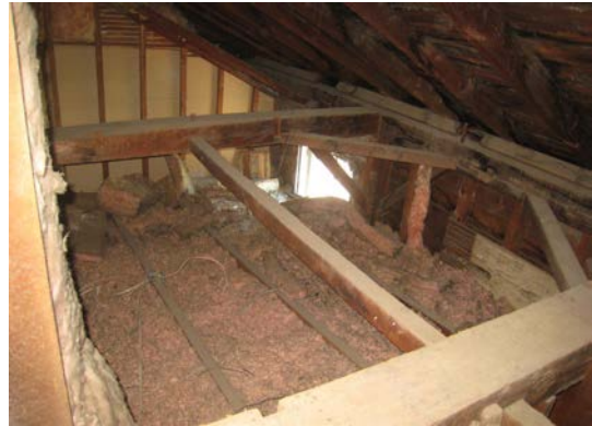
Attic and roof framing over the assembly room.
