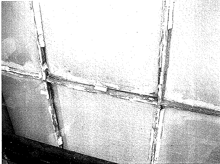
FIRST FLOOR WINDOW SOUTH ELEVATION • Broken / Missing Glazing Putty
