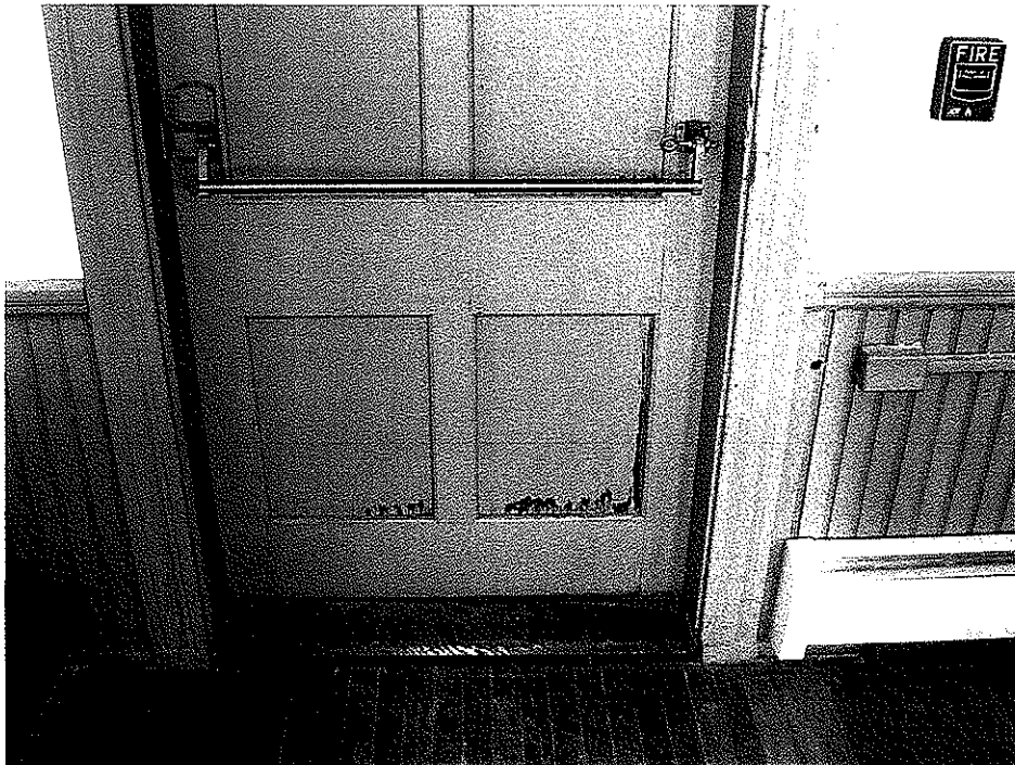
SECOND FLOOR FIRE ESCAPE EXIT DOOR
