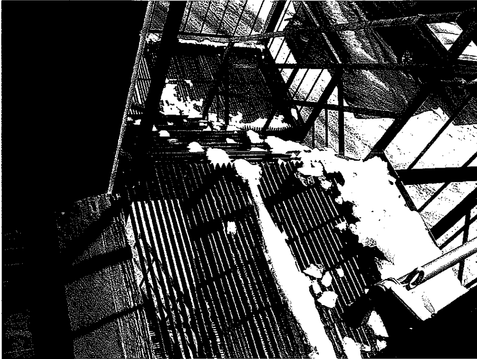
SECOND FLOOR FIRE ESCAPE
