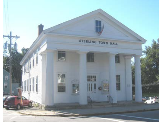
The facade (north elevation).
