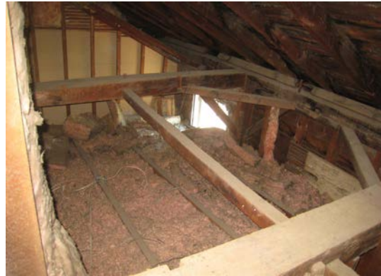
Attic and roof framing over the assembly room.
