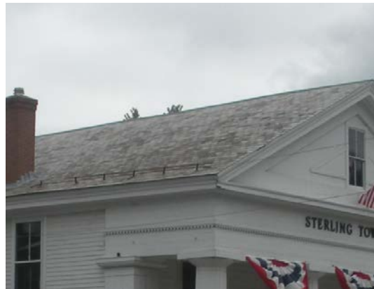
Snow rail and chimney flashing at slate roof.
