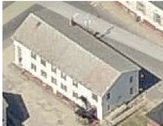
Aerial view of roof from south west. (Image from Bing.com)
