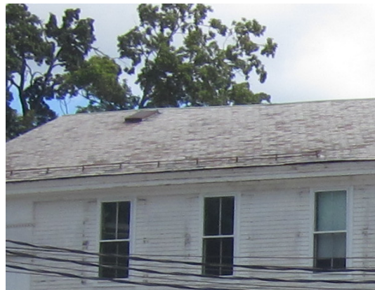
Snow rail and roof hatch on slate roof.
